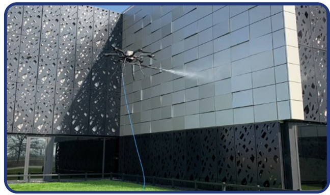
Cladding cleaning with Wash Drones
