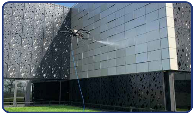
Cladding cleaning with Wash Drones
