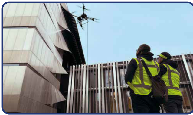
Cleaning buildings constructed under architecture with Wash Drones
